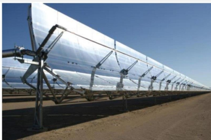
Figure 2.6: Parabolic trough concentrator
